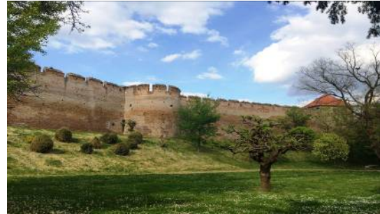
2nd south side - part of walls; TB Ilok
