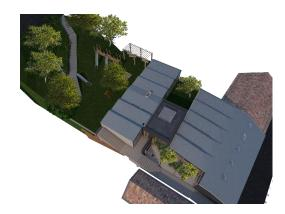
**Materials:** Foundations, walls and columns are made of reinforced concrete. Folded roof and pitched roof are made of CLT (timber).
