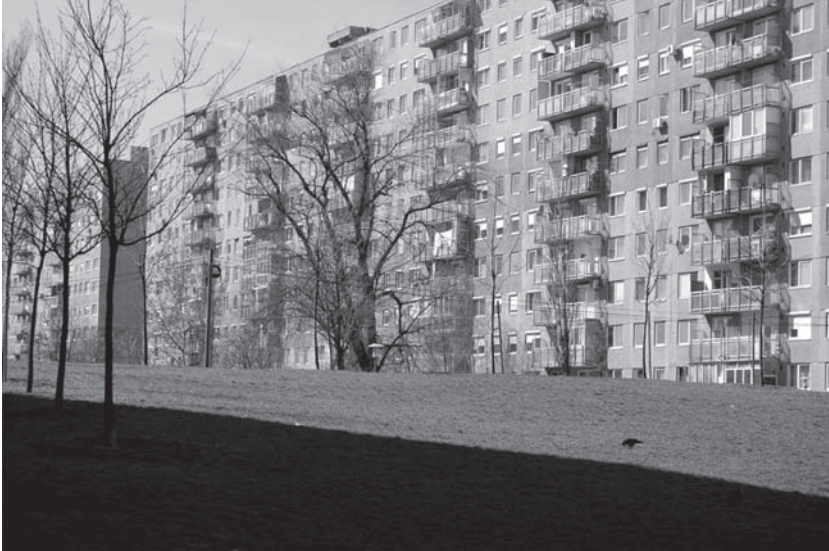
Figure 6. Havana Housing Estate, Budapest, 2014. (Author's photo.)
