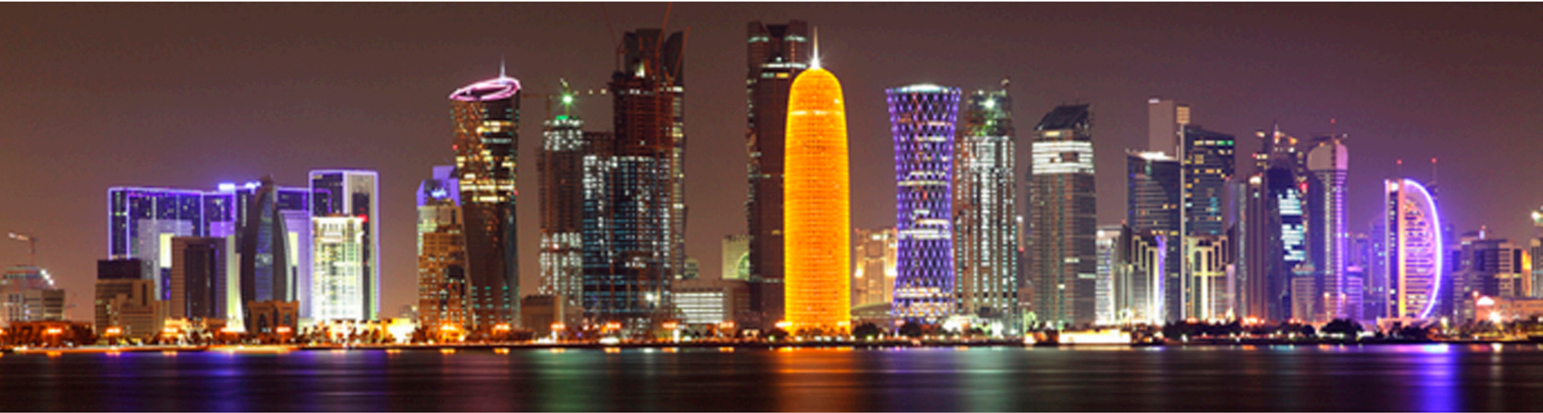
Skyline of the city of Doha, Qatar
